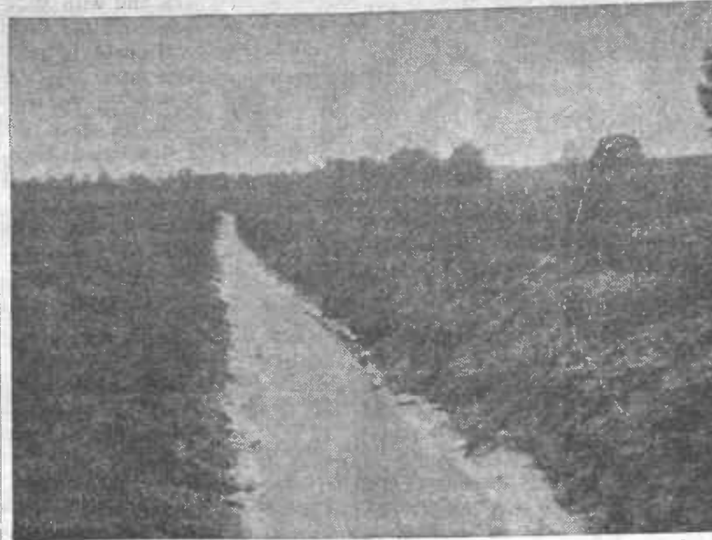
DRAINAGE DITCH — A small dragline drainage ditch on Omar Epps farm, 2 miles north of Tishomingo on Highway 25, is a good example of proper land drainage for better crop yields. (Soil Conservation Service Photo)
